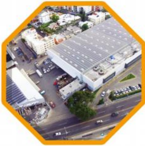
FERRETERIA BELLON 850 kW
